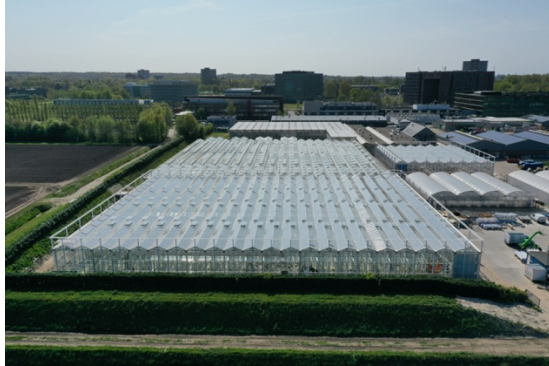
Photo caption: Construction of the Serre Red research greenhouse nears completion at Wageningen campus (April 2020, photo courtesy of Unifarm – Wageningen University & Research)
